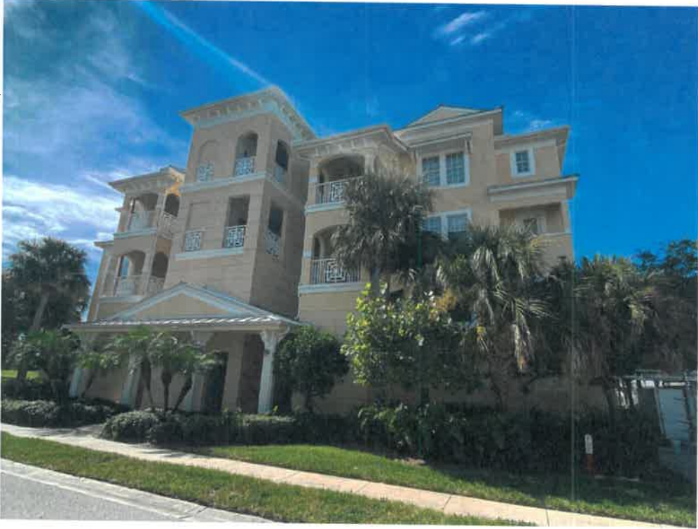
Figure 1: Typical 4-Story Roof Type (Metal) and Geometry (Hip)
